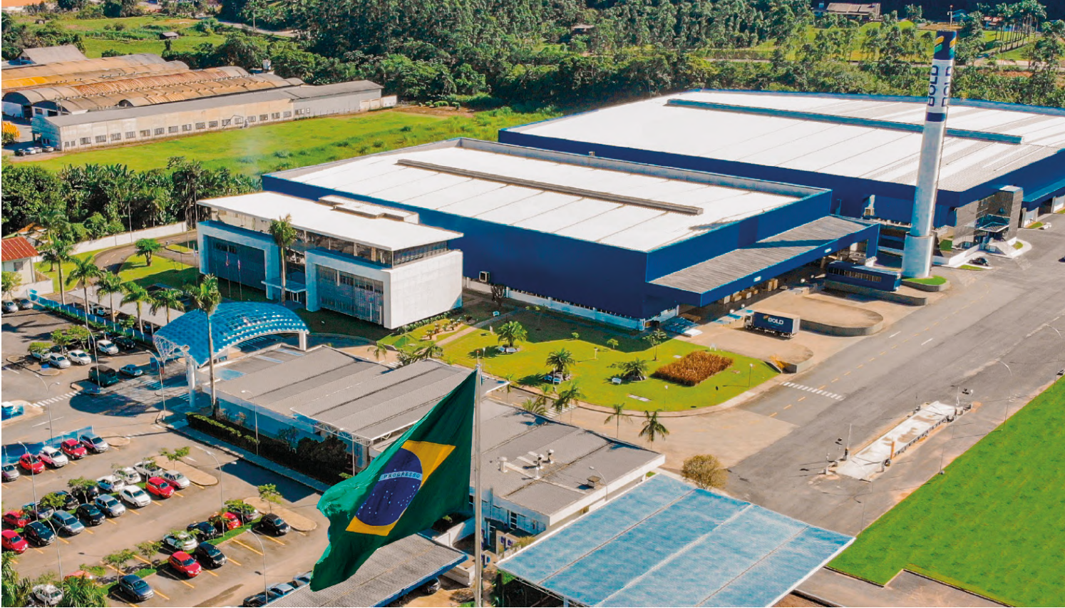
Headquarters in Jaraguá do Sul / Santa Catarina.
